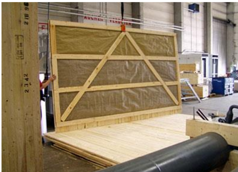
Figure 6: Side wall lined with a barrier layer
